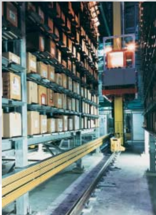
13 pole multipole conductor rail with double current collectors in the high bay storage of a warehouse.
